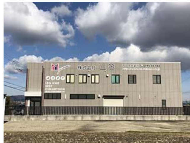
Nara Office/ Distribution Center
